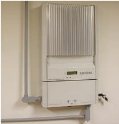
Figure 8: Grid-Tie PV Inverter Installation
