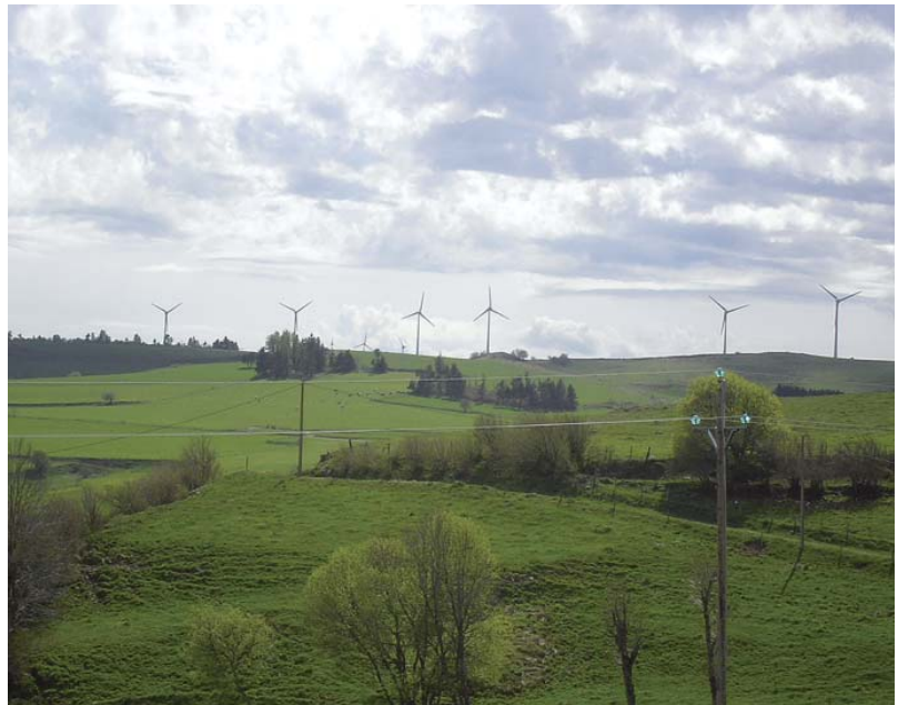
Le Saulzet E-48 wind farm (Puy-de-Dôme) in May, situated at 1,200 metres above sea level.
